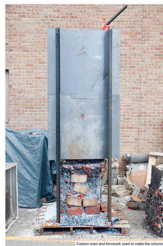
Custom oven and formwork used to make the columns
